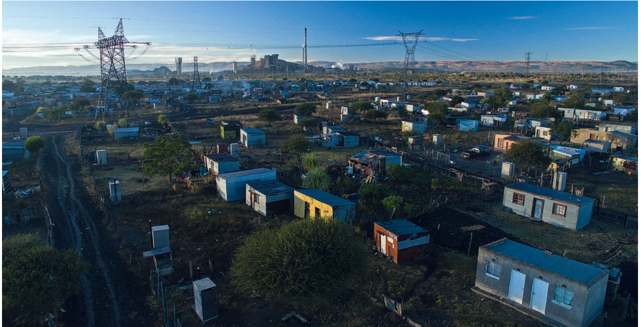
Settlements extending upto the powerlines, but there is no electricity for shackdwellers in Wonderkop.
