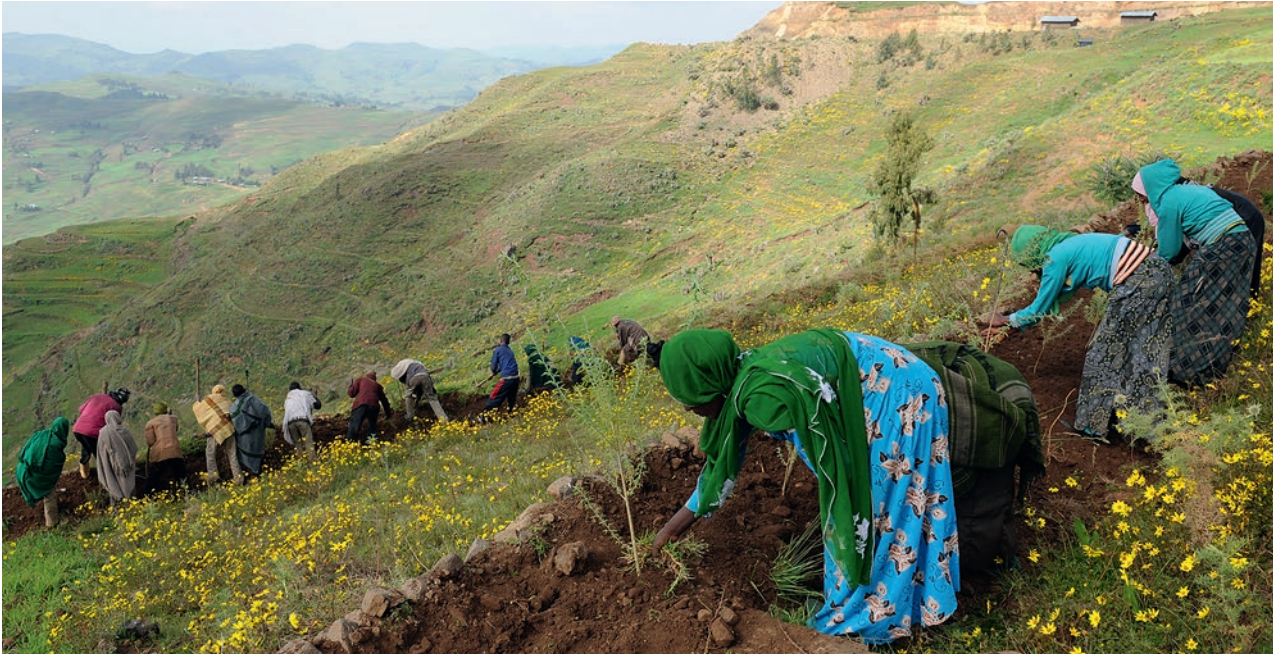
In sweeping community work, the residents of Chulke in the highlands of Ethiopia erected terraces and stone walls, that the area doesn't further degrade. Behind it, soil was piled up and planted with seedlings of trees.
