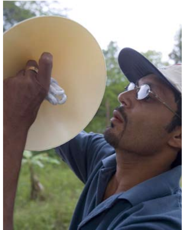
Electrician Wasanthe from project partner ASPIRA in Sri Lanka fits a low-energy light bulb (compact fluorescent lamp, CFL) into a streetlamp. Photo: Paul Hahn
