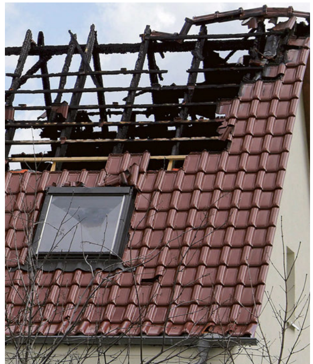
Proposed housing for migrants in Germany which was set on fire by right-wing extremists to disrupt placement of migrants.
